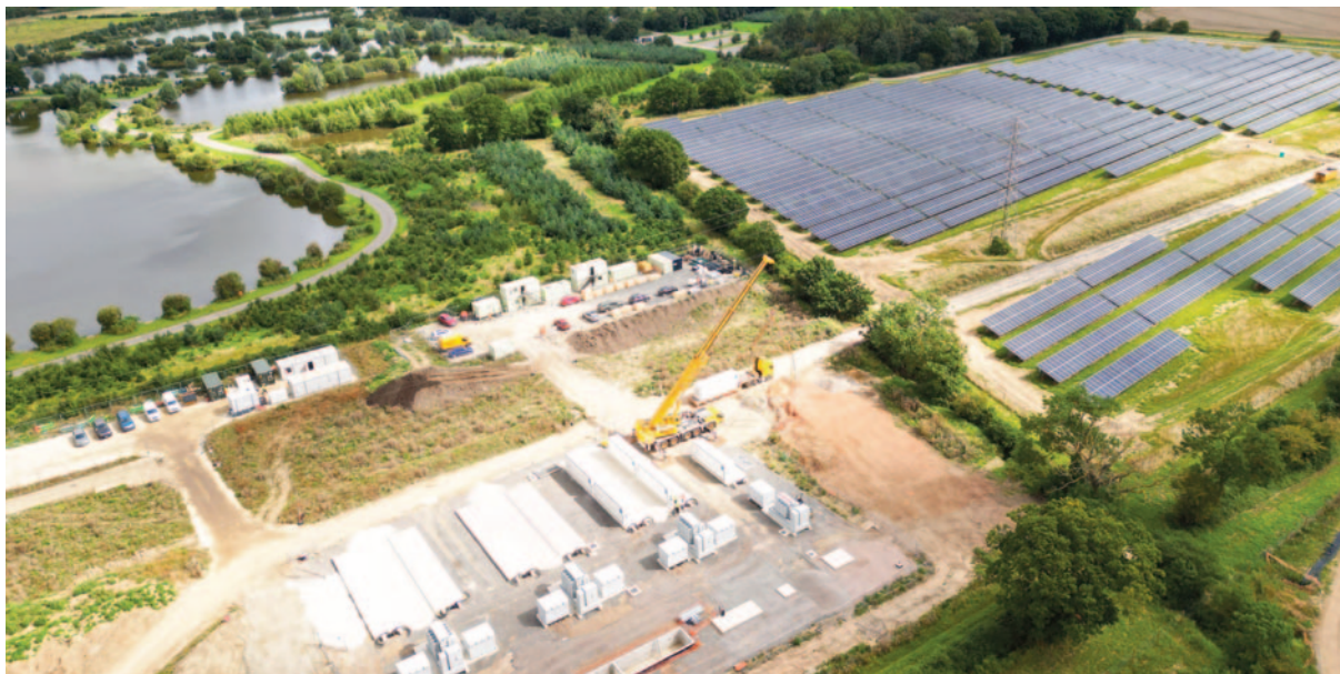
Tiln solar park, 61 MW PV coupled with 25 MW / 50 MWh BESS. Retford, England.
