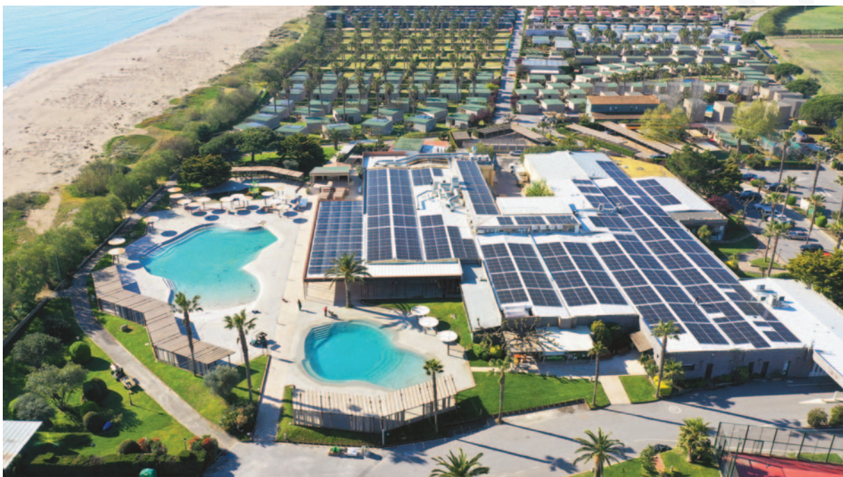
Rooftop PV system with 234 kWh BESS in Girona, Spain.
