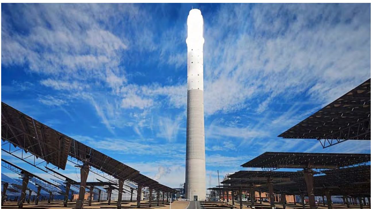
"Noor III Ouarzazate CSP Plant, Morocco"
